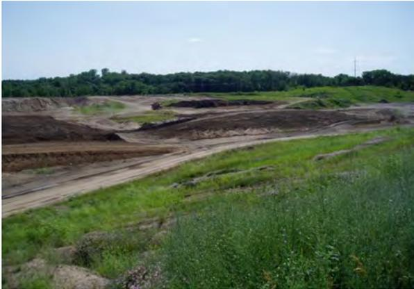
**Lot benching** is often utilized in subdivision developments. Lots are strategically graded to direct the runoff from each lot to a stable outlet rather than to an adjacent lot. Lot benching can result in reduced slope lengths and steepness, decreasing the potential for soil erosion. Lot benching establishes drainage patterns early in the construction process for each lot therefore avoiding potential drainage problems in the future when home construction begins.
