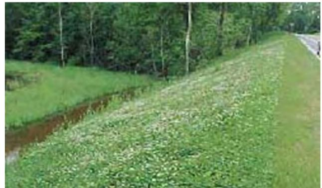
The permanent stormwater treatment system must be in place and functioning. Drainage ditches and other conveyance systems must have all collected sediment cleaned out and be stabilized with permanent cover. Temporary erosion and sediment control BMPs must be removed.
